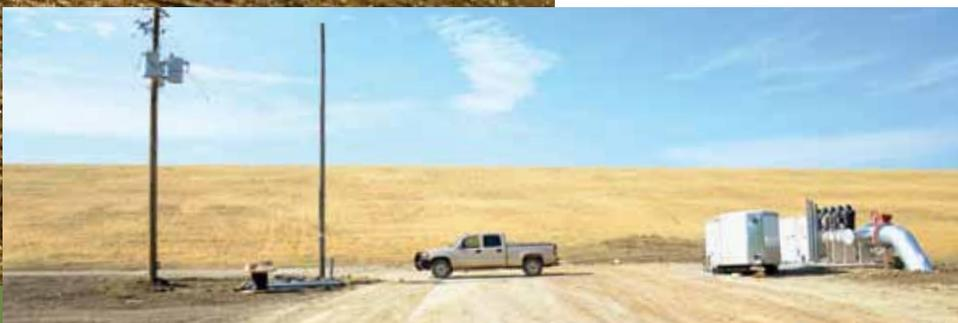
*New utility poles and lines power a pumping station, where five high-efficiency electric motors deliver water to the center pivots. Dwarfing them all is the 45-foot-tall dam holding back the new reservoir.*
